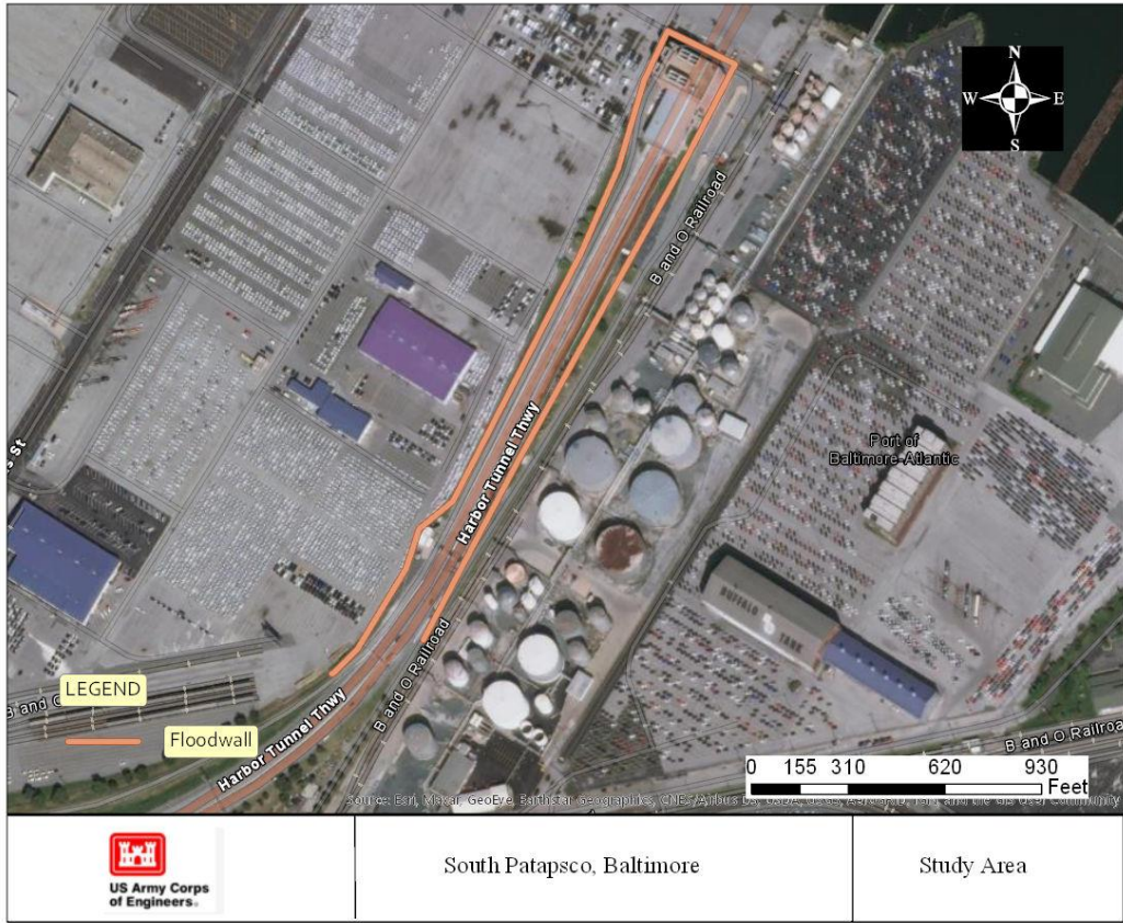
Figure 4, Study Area- 895 Tunnel and Ventilation Building
